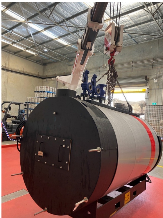
Crane lift of boiler vessel into facility during installation
